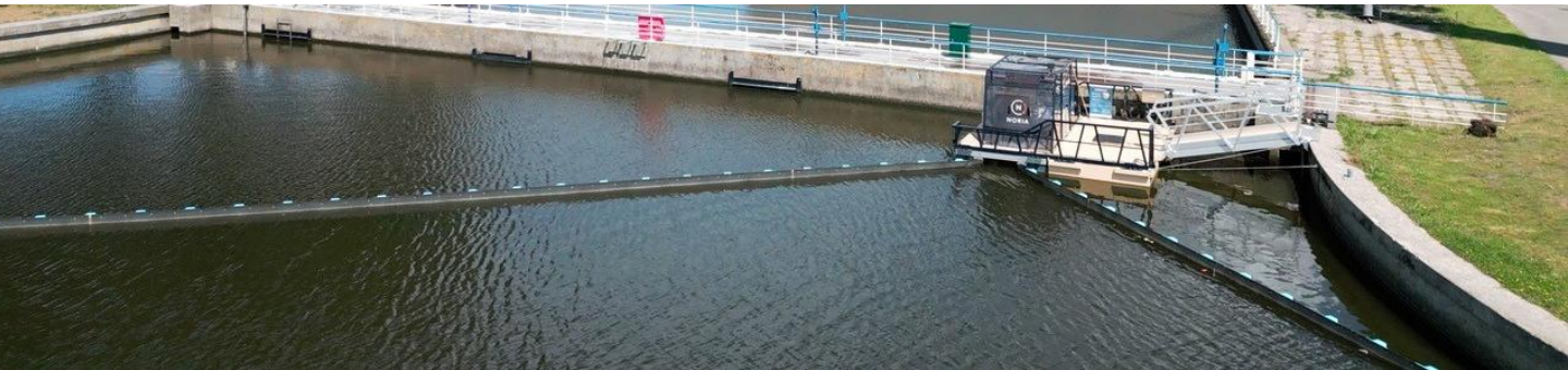
The Noria CirCleaner in Den Helder. Two floating lines guide the litter towards the system.
